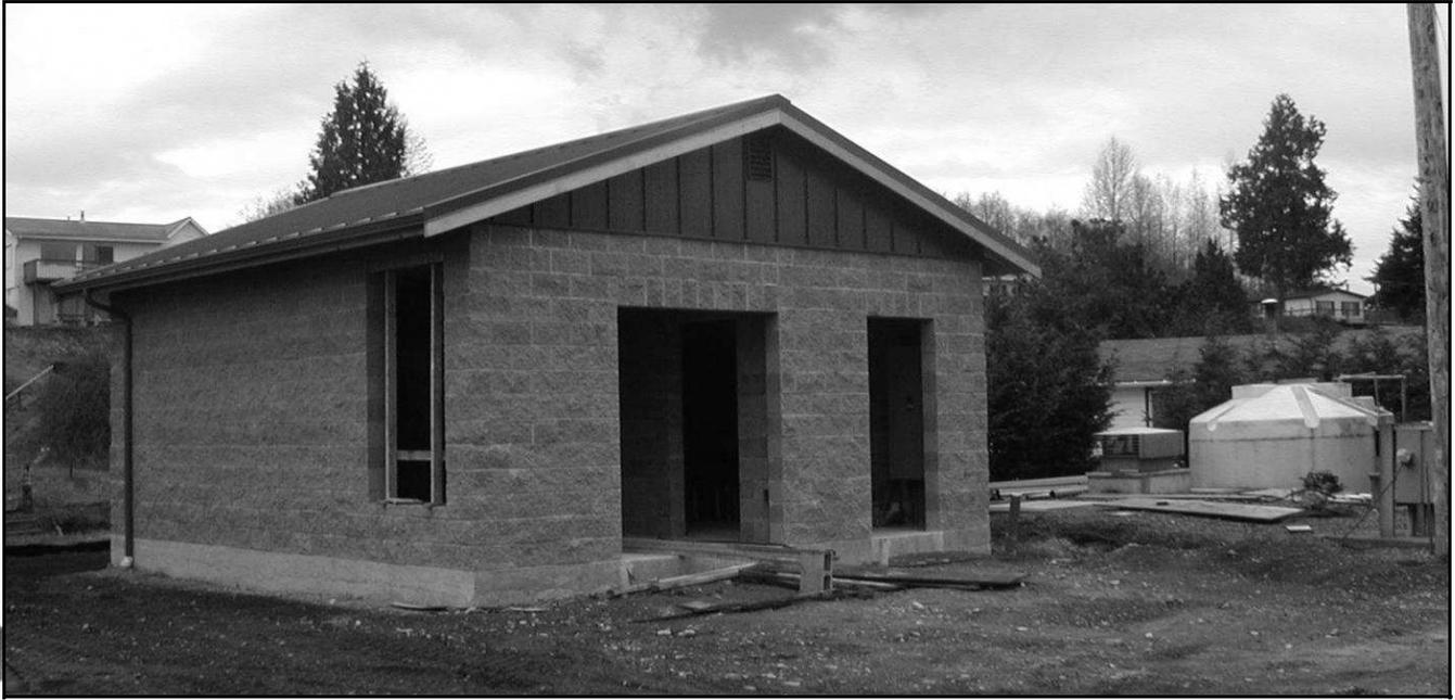
The District is currently working on Pump Station #3 Rehabilitation. This pump station, located near Birch Bay Drive and Maple Street, is the District's main station for pumping sanitary wastewater to the Treatment Plant. This project will replace the existing below ground station with the building shown above and increase pumping capacity by approximately 30%
